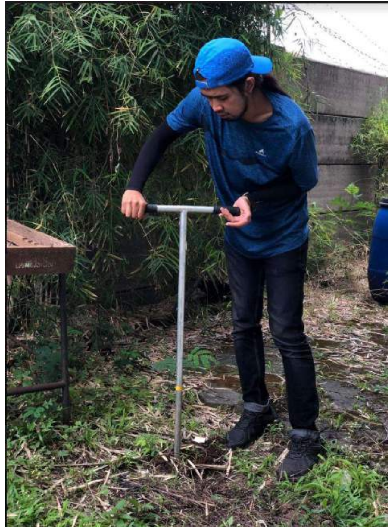
Preparation of Rainwater Harvesting
