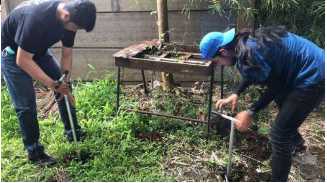
Building SWG in Bandung areas
