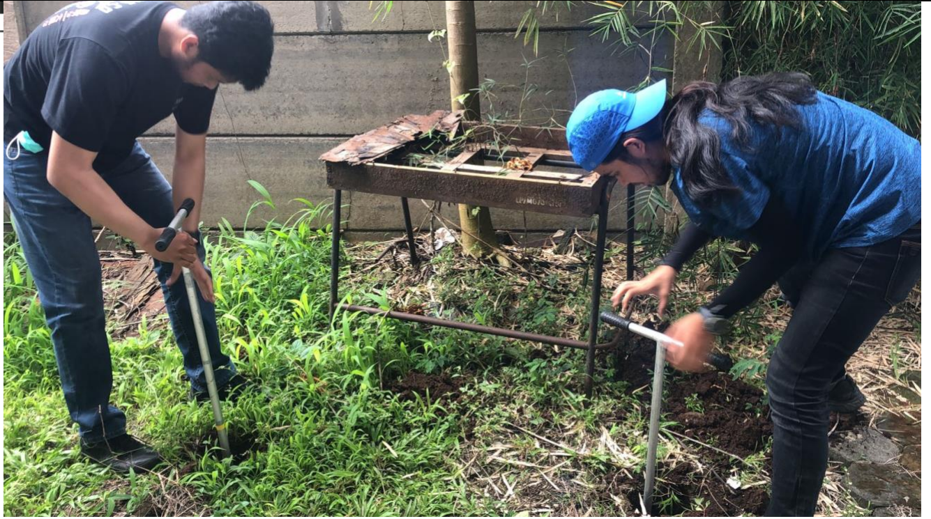
Building SWG in Bandung areas
