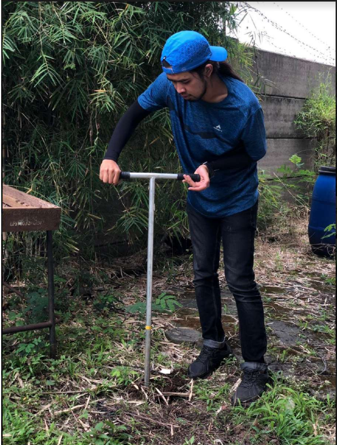
Preparation of Rainwater Harvesting
